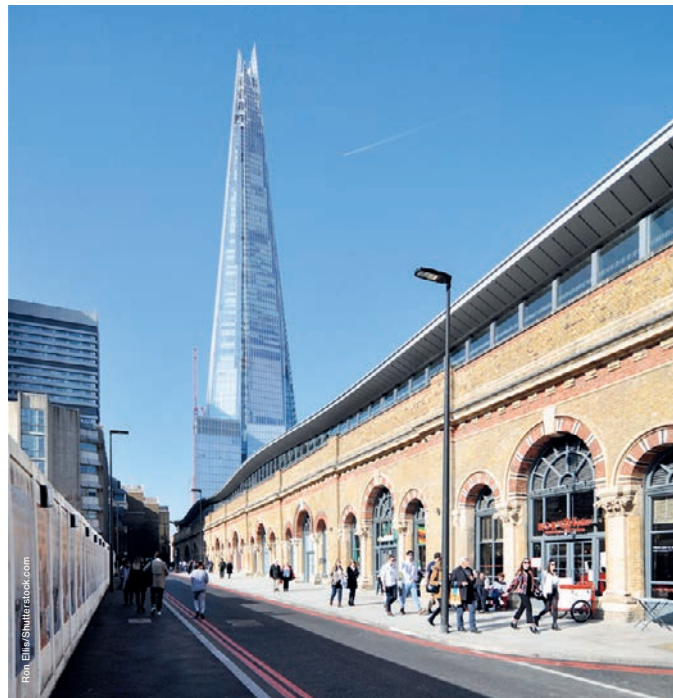
London Bridge Railway Arches
